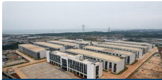
Hydrometallurgy production base in Leizhou City, Guangdong Province
